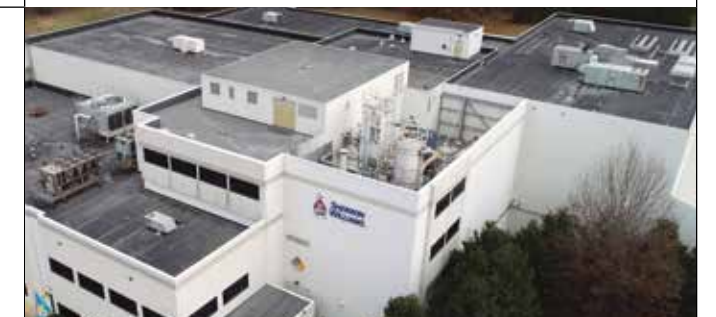
Charlotte Manufacturing Plant - Before
