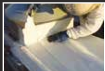
EMBEDDING REINFORCEMENT FABRIC AROUND DETAILED AREA
