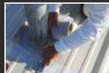
APPLYING SEAM TAPE AROUND PENETRATION AREA
