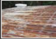
HEAVILY OXIDIZED METAL ROOF
