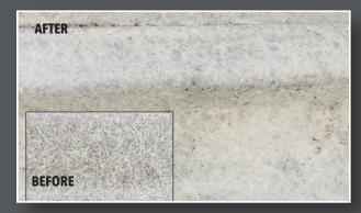
Cleaning assists in eliminating raised reinforcement fibers and provides a clean and smooth surface ready for application.
