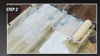
**Apply** KST Roofing Solutions<sup>™</sup> Skylight<sup>™</sup> Restoration Coating to fiberglass skylight to help improve light value within building structure.
