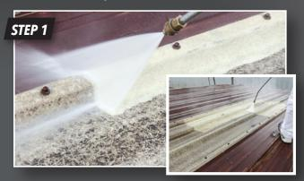
**CLEAN** fiberglass to remove weathered reinforcement fibers and prepare surface for KST Roofing Solutions™ Skylight™ Restoration Coating application.
