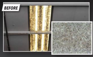
**Fiberglass skylight BEFORE.** Raised reinforcement fibers indicate age. Restore with KST Roofing Solutions™ Skylight™ Restoration Coating.
